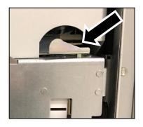
Fig. 243: Contactor truck locked
