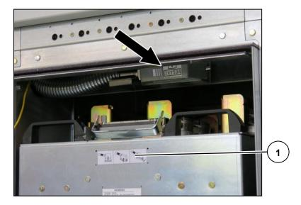
Fig. 340: Low-voltage connector stowed away
