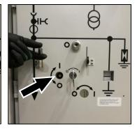
Fig. 192: Lifting the operating Fig. 193: Turning the double-bit key counter-clockwise
