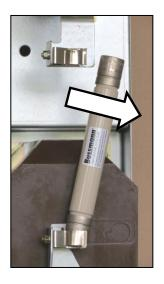
Fig. 171: Pulling off the fuse-link
