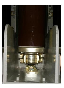
Fig. 260: HV HRC fuse-link inserted and fuse-link bracket closed on the opposite side of striker area
