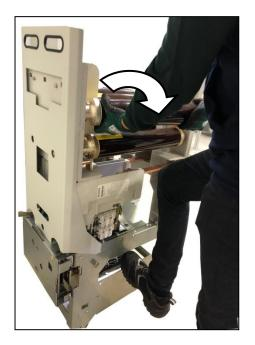
Fig. 247: Opening the fuse-link bracket in the striker area (operating side of contactor truck)
