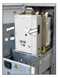
Fig. 120: Pulling out the withdrawable circuit-breaker type 3AE5
