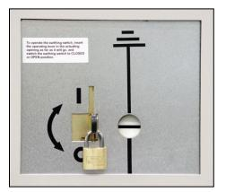
Fig. 522: Operating slide on busbar earthing switch padlocked
