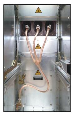
Fig. 685: Earthing device completely mounted
