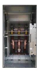
Fig. 554: Switch-disconnector panel only: Switching-device / connection compartment accessible
