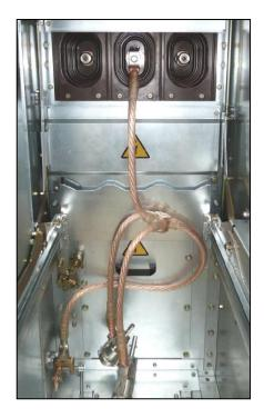
Fig. 684: Earthing tulip fixed on central bushing contact
