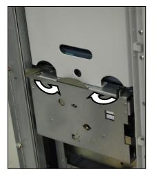
Fig. 242: Interlocking the contactor truck
