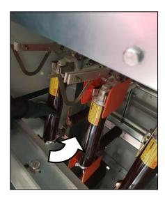
Fig. 422: HV HRC fuse-link inserted on the opposite side of striker area
