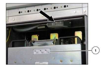
Fig. 314: Low-voltage connector stowed away
