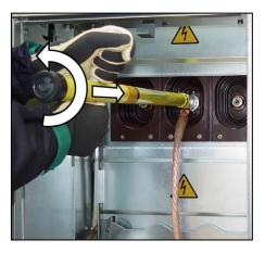
Fig. 689: Detaching the earthing tulip
