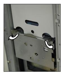
Fig. 227: Releasing the interlocking with the panel
