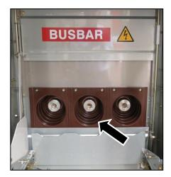
Fig. 532: Shutter to the connection compartment open
