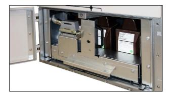
Fig. 426: Door to the voltage transformer compartment open
