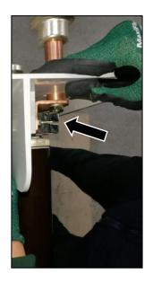
Fig. 250: HV HRC fuse-link removed on the opposite side of the striker area
