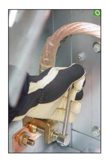
Fig. 692: Earthing clamp connected with earthing point
