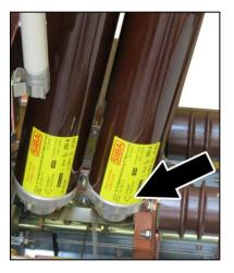
Fig. 351: Striker pin pointing to lower clamp
