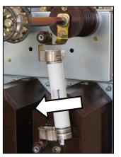
Fig. 177: Pushing the lower end into the clamp
