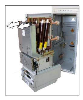
Fig. 322: Pulling the contactor truck
