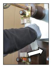
Fig. 175: Pulling off the fuse-link
