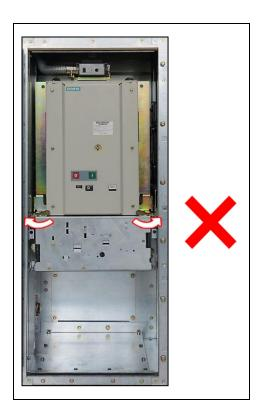
Fig. 114: Circuit-breaker panel without service truck
