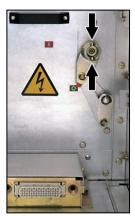
Fig. 236: Coupling in the switching-device compartment
