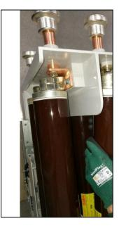
Fig. 254: HV HRC fuse-link inserted and fuse-link bracket closed on the opposite side of striker area
