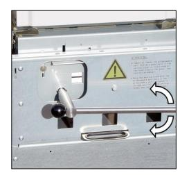
Fig. 130: Operating the feeder earthing switch operating shaft
