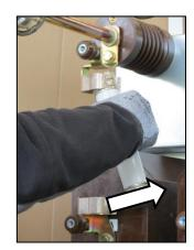
Fig. 372: Pulling off the fuse-link
