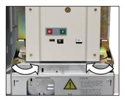
Fig. 121: Interlocking the withdrawable circuit-breaker
