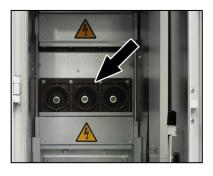
Fig. 547: Shutter to the connection compartment open
