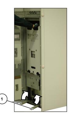
Fig. 240: Pushing the contactor truck at the top into the panel
