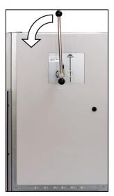
Fig. 518: Opening the busbar earthing switch
