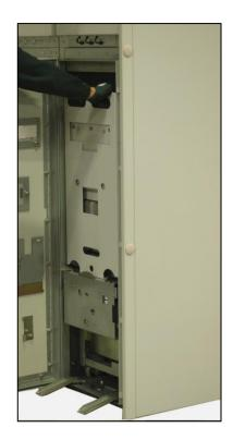
Fig. 230: Moving the contactor truck using two handles
