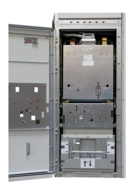
Fig. 318: Panel front with open high-voltage door
