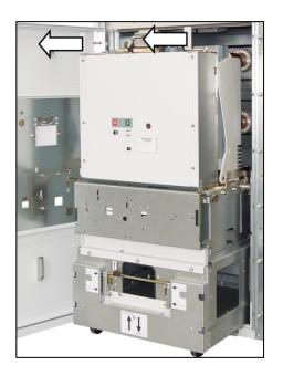
Fig. 148: Pulling out the circuit-breaker truck
