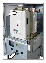
Fig. 136: Pushing the withdrawable circuit-breaker into the panel
