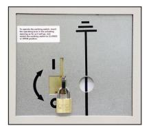
Fig. 509: Operating slide on busbar earthing switch padlocked
