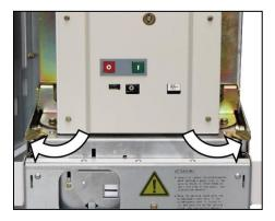
Fig. 134: Releasing the interlocking of the withdrawable circuit-breaker
