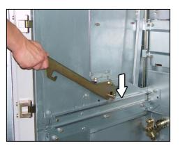
Fig. 525: Pushing on the slip-on lever
