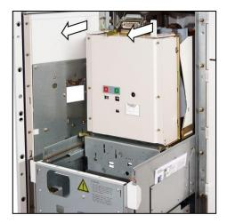
Fig. 119: Pulling out the withdrawable circuit-breaker type 3AE1
