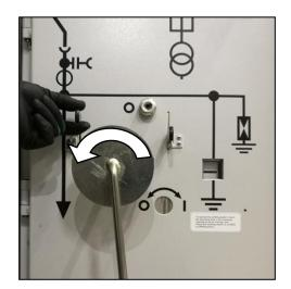
Fig. 209: Turning the racking crank counter-clockwise
