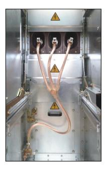
Fig. 686: Earthing device to be removed
