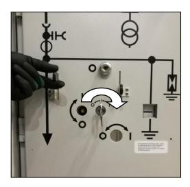
Fig. 189: Turning the double-bit key clockwise
