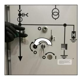
Fig. 196: Turning the double-bit key counter-clockwise
