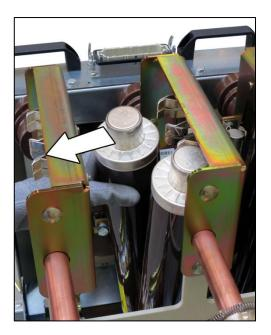
Fig. 350: Removing HV HRC fuse-links from the middle phase
