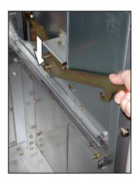
Fig. 530: Pushing on the slip-on lever
