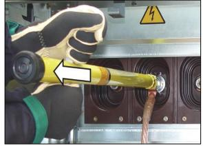
Fig. 683: Detaching earthing rod
