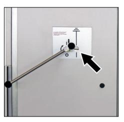
Fig. 521: Operating lever in end position
