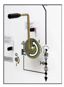
Fig. 72: Turning the racking crank counter-clockwise
