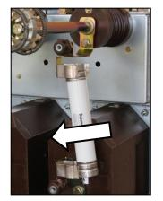
Fig. 374: Pushing the lower end into the clamp
