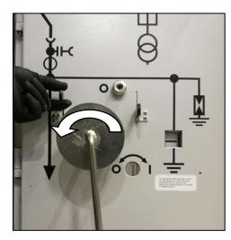
Fig. 195: Turning the racking crank counter-clockwise
