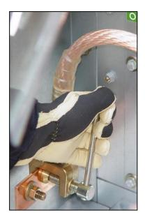
Fig. 677: Bolting earthing clamp
