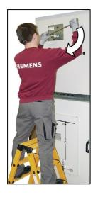
Fig. 505: Closing the busbar earthing switch Fig. 506: Closing the busbar earthing switch using an electrician's ladder
