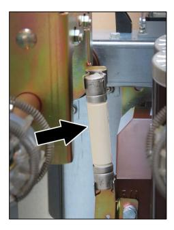
Fig. 361: First protection fuse-link replaced
