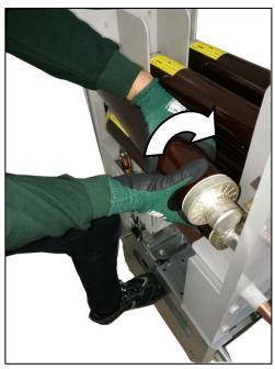
Fig. 251: Inserting the HV HRC fuse-link in the striker area
