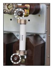
Fig. 173: Insulating cover removed
