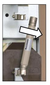
Fig. 368: Pulling off the fuse-link
