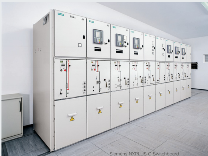
Siemens NXPLUS C Switchboard
