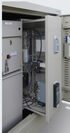
Class B RMU in Bosecker enclosure with pull-out drawer
